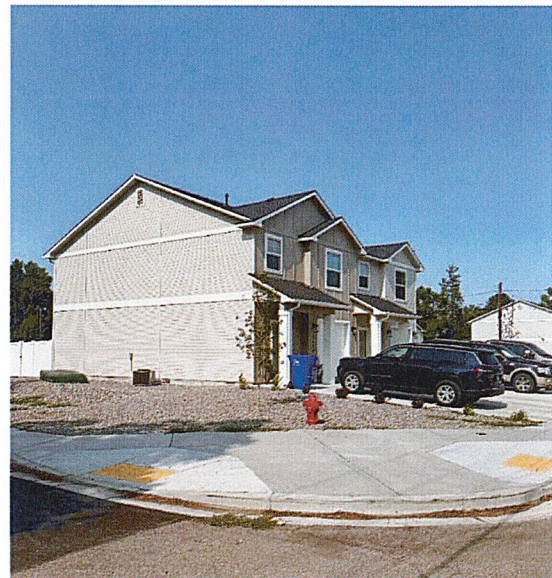
Image 3. Duplex dwelling units in New Plymouth.
