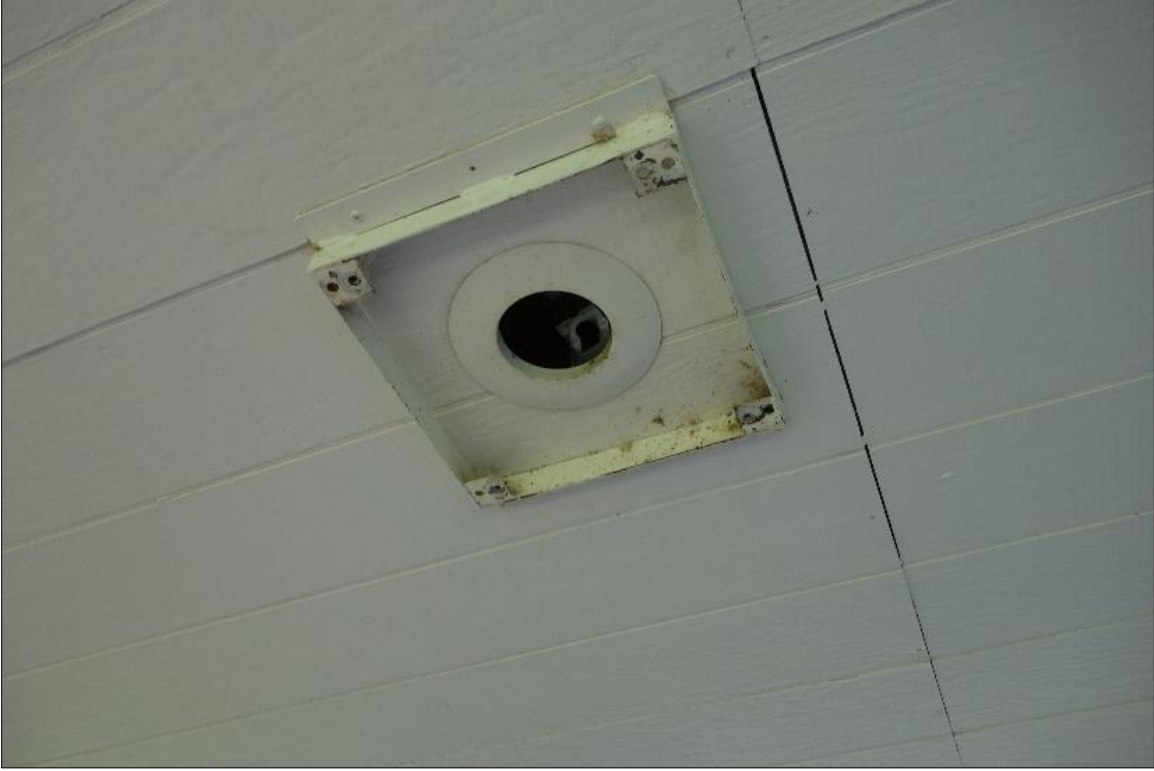
Missing Lighting in Pavilion
