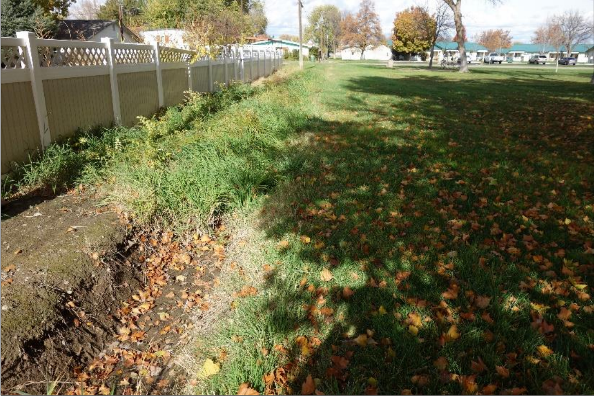
Grass Filled Ditch
