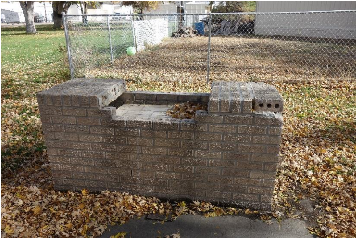
Fire Pit to Be Removed
