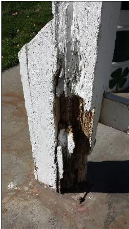
Pavilion Support In Poor Condition
